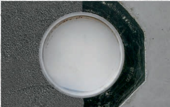
Concreted UFR with PMBC
