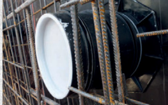
UFR in formwork
